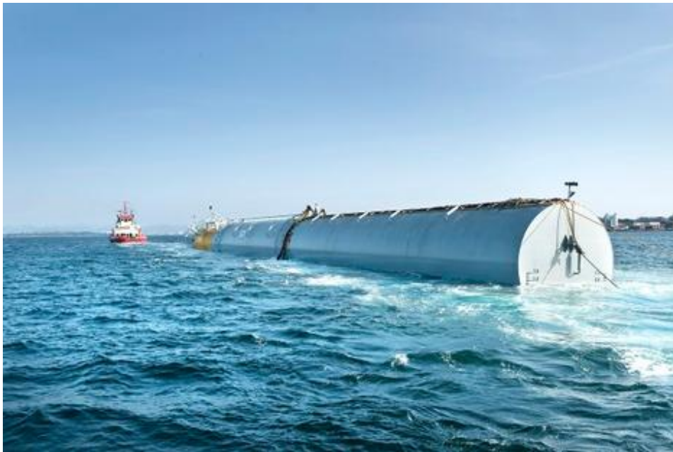
Figure 2. Wet towing of a FTWU substructure. 8
