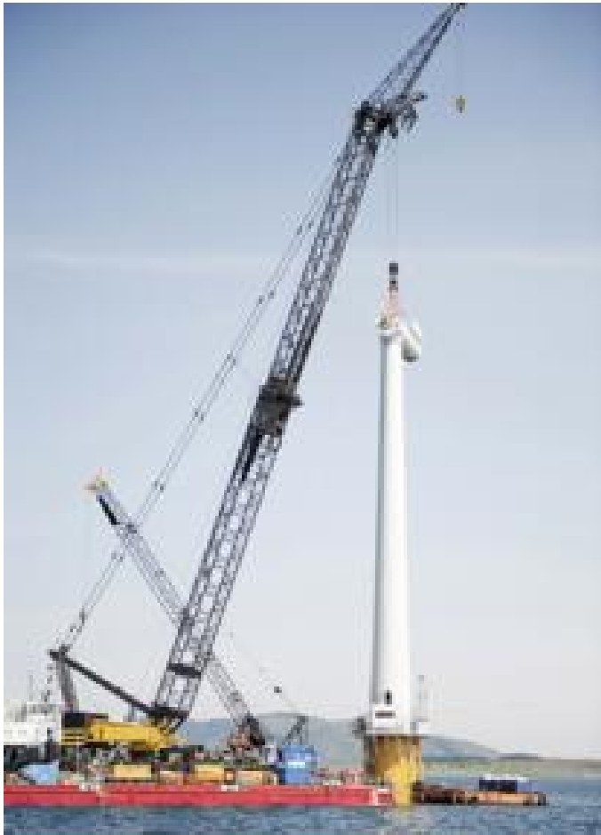
Figure 4. Assembling a nacelle by a Crane Vessel.
