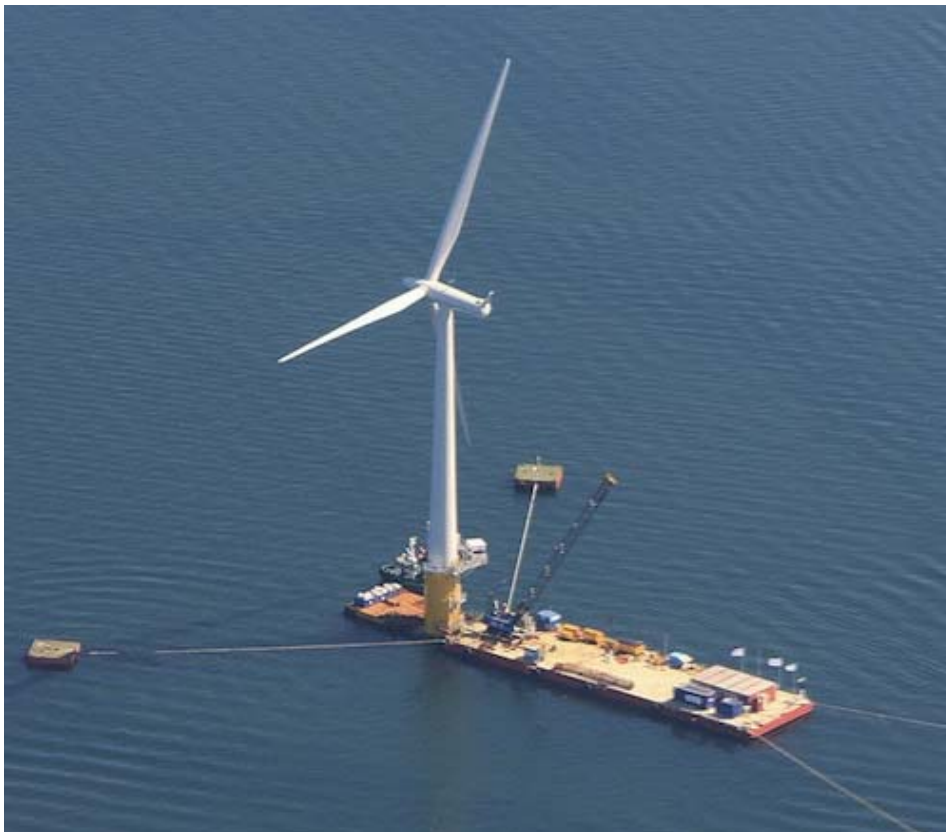
Figure 3. Anchoring and Hook-up operations. 8
